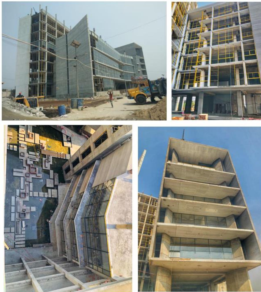
Current Status of Construction work in Photos
